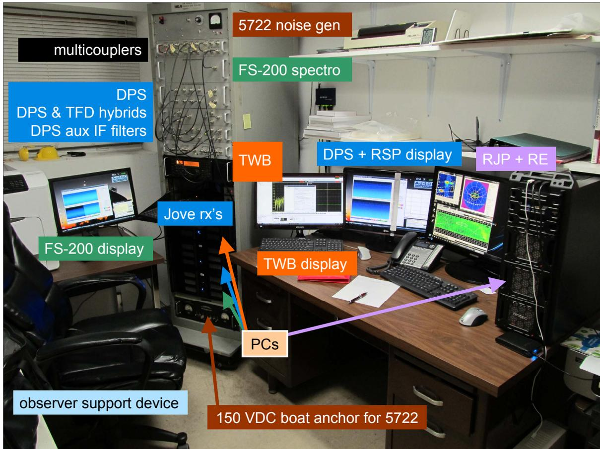
DPS installed in a 19" rack. AJ4CO Observatory, High Springs, Florida.
