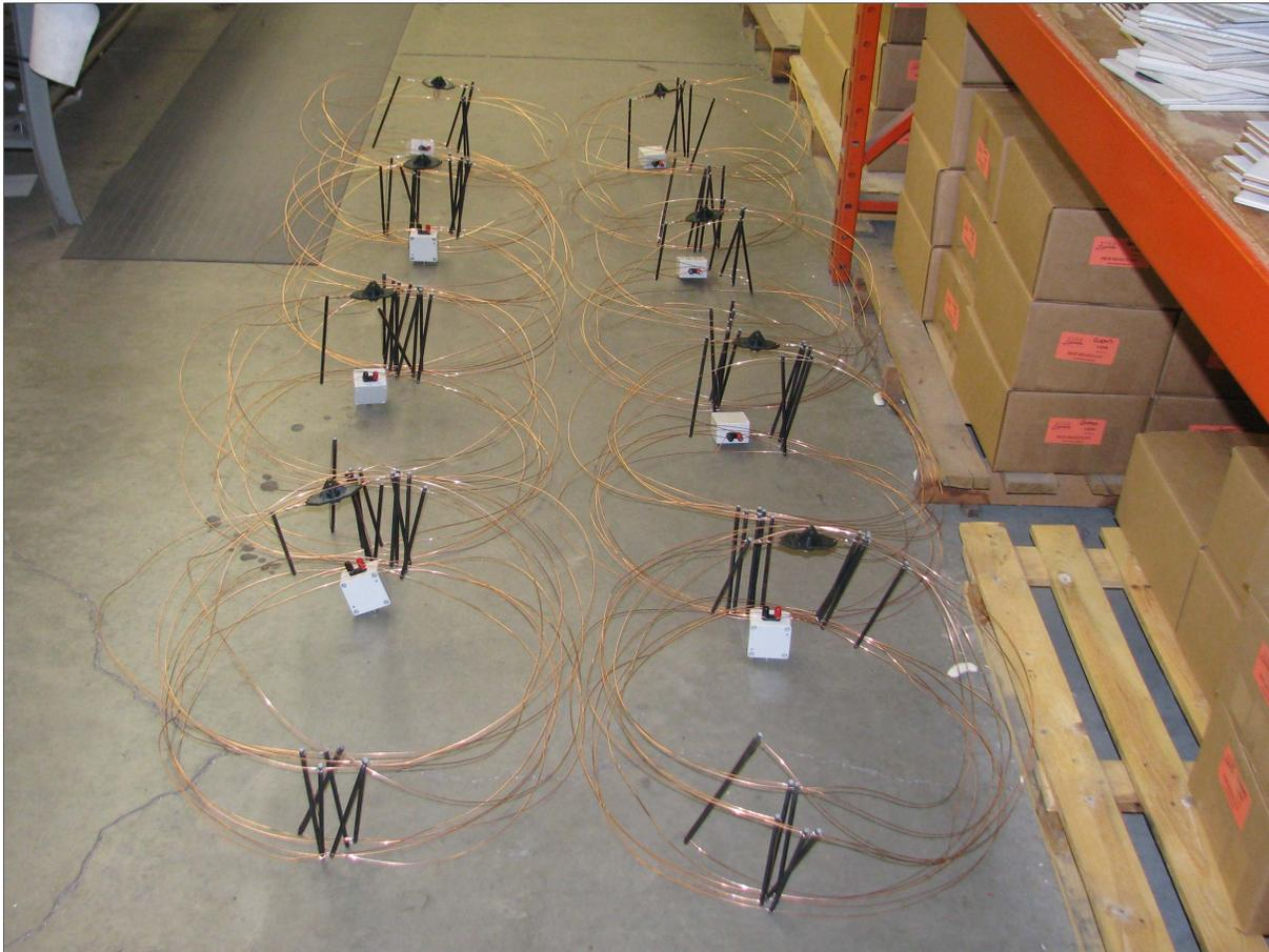
Eight TFD elements ready for installation. This represents 500 feet of 16 ga Copperweld (about 62 feet per element).
