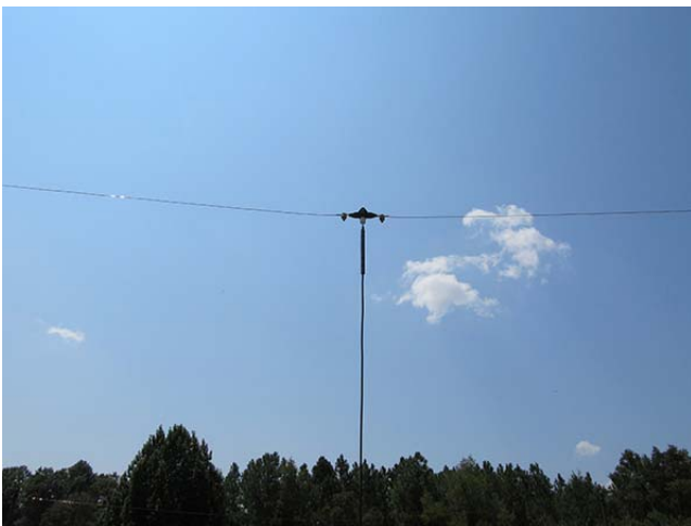
Feed point after element installation.
