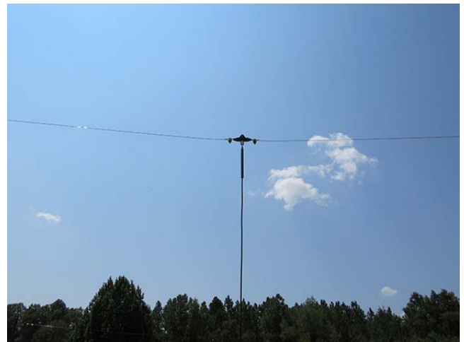
Feed point after element installation.
